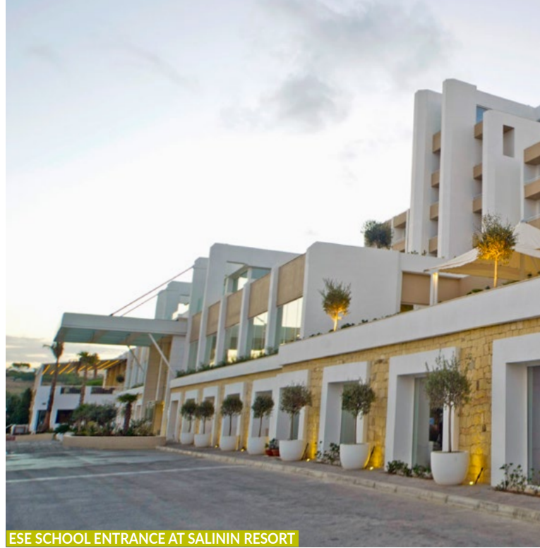
ESE SCHOOL ENTRANCE AT SALINI RESORT
